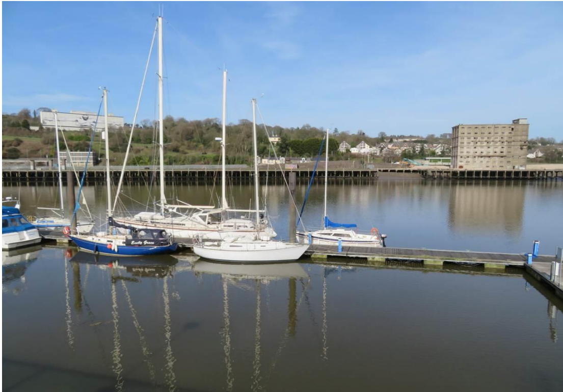
Plate 11.3 View from Meagher's Quay north along the route of the proposed bridge towards the North Quays, showing derelict industrial building on wharf to right of photo, with the former Ard Rí Hotel (left horizon) and Sion Hill House (centre) on Mount Sion to the rear. Housing developments in the Ferrybank neighbourhood are also visible in the right background. (View B from Plate 11.1)
