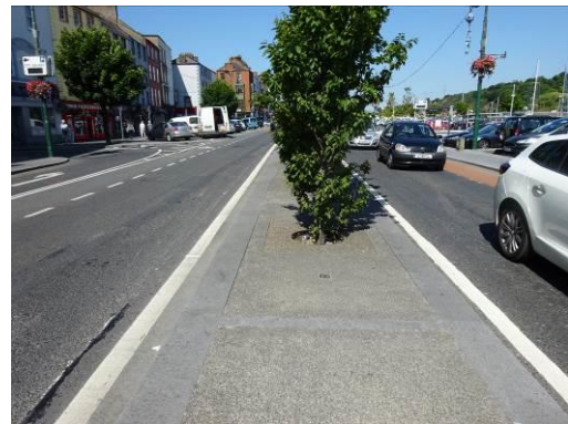
Plate 5.6: Planted Median along R680
