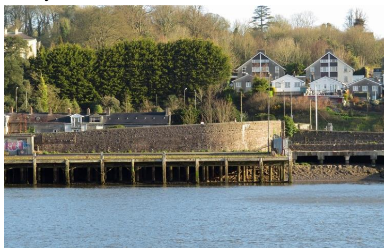
Plate 15.11: Site for bridge landing at Ferrybank
